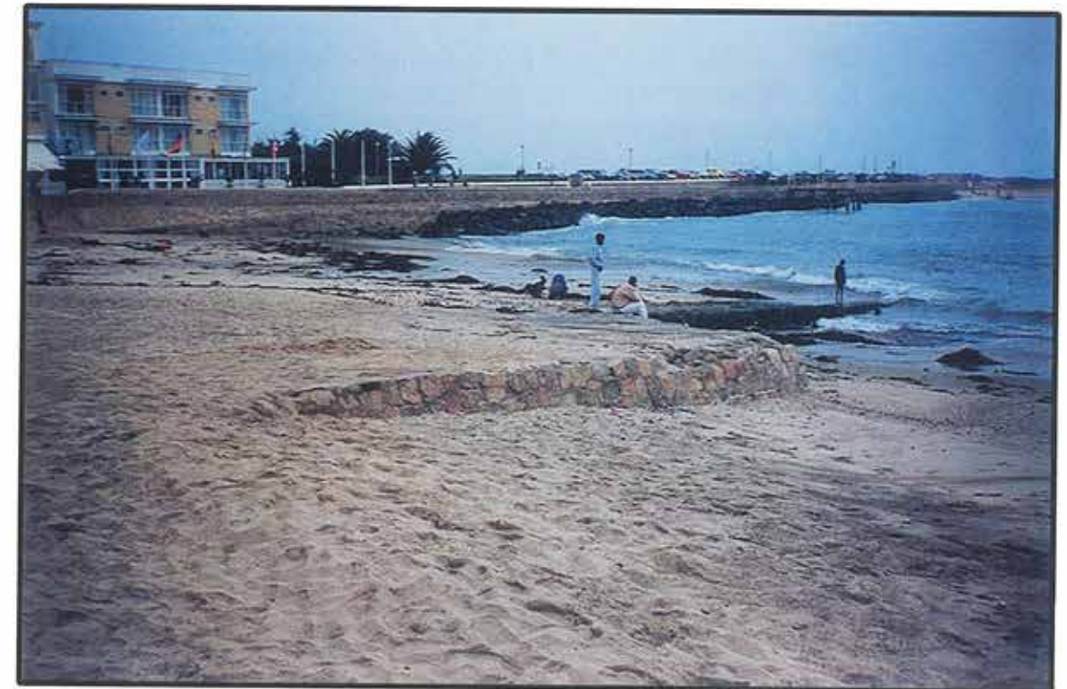
Plate 4: Example of severe beach erosion at The Mole in Swakopmund. The old slipway is now visible in the foreground (June 1997).
